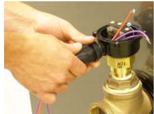
Fig. 5 - Flow Switch Wiring
