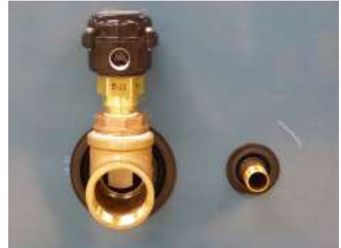
Fig. 4 - Final Flow Switch Position
