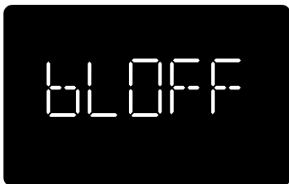
Figure 17 - Follower Homescreen 2 - Boiler Off
