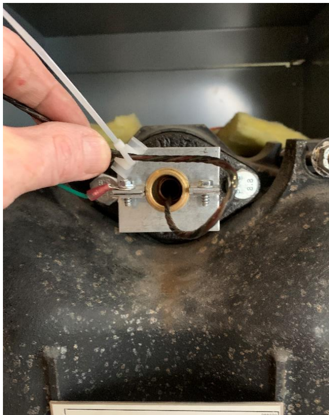
New Well and probe installed
