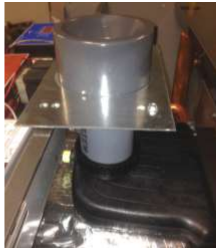
Figure 7 – Installation of New Flue Adapter
