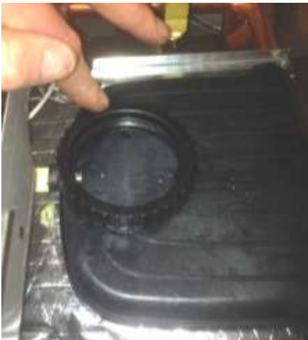
Figure 6 – Installation of New Flue Gasket
