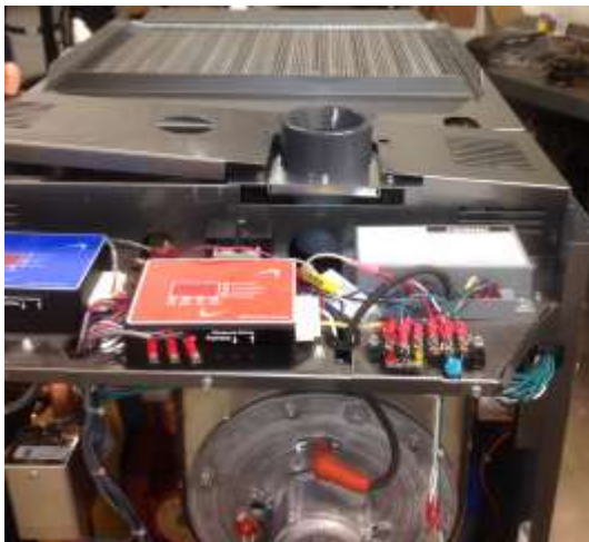
Figure 8 – Reinstallation of Middle Top
