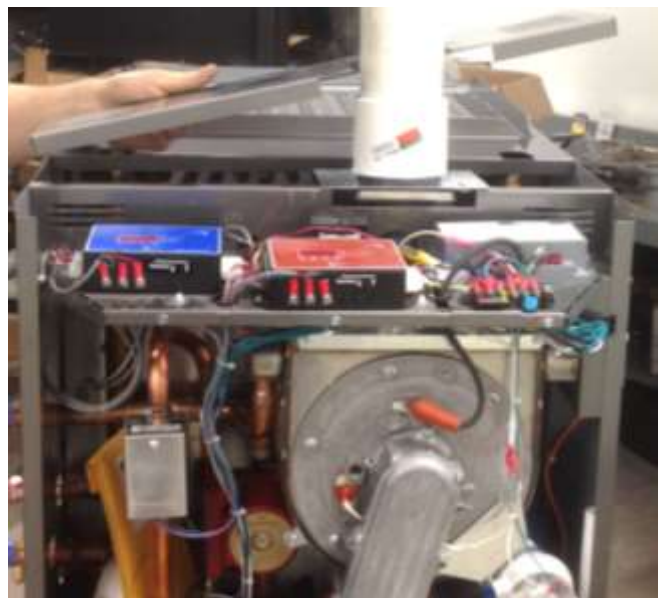
Figure 3 – Removal of Middle Top
