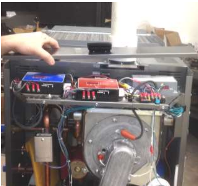
Figure 2 – Removal of Front Top
