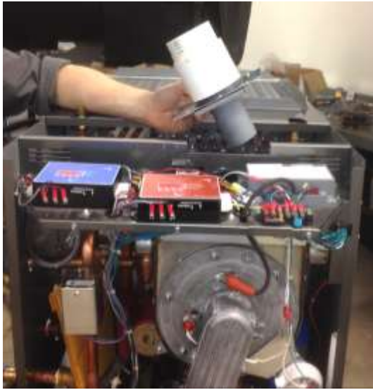
Figure 4 – Removal of Old Flue Adapter
