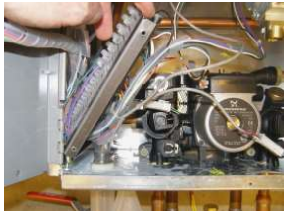
Moving Wiring Terminal Strip
