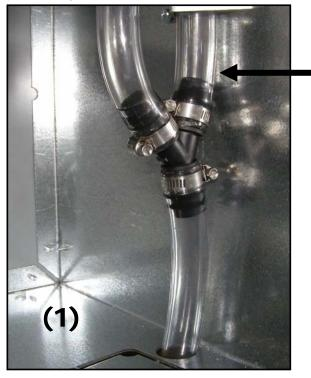
**<u>CAUTION:</u>** Do not cut or pull on this tube. It must remain connected to the boiler.
